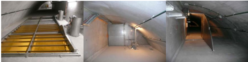
Figure 4: Fresh-air impulse device: damper (left), blocking element closed (centre), blocking element open (right)
